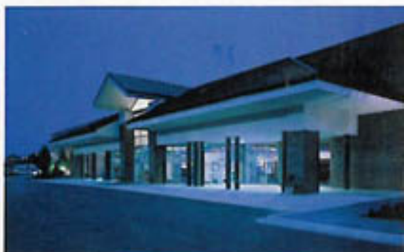
Abt, established in 1936, has been providing the customers in the Chicago land area with the finest appliances and audio/video equipment for more than 70 years.
